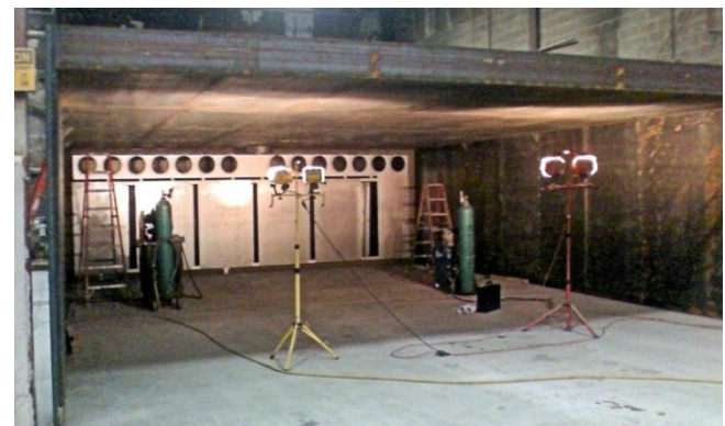
The oven in the process of being installed at CCPI
